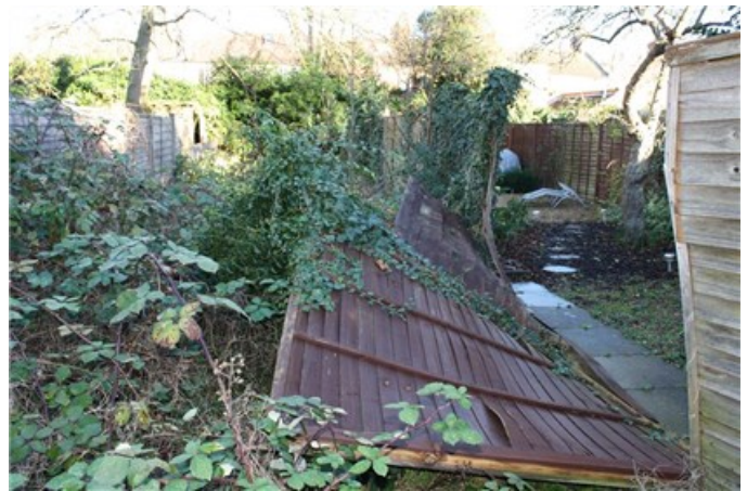
Rear garden - fence collapsed
