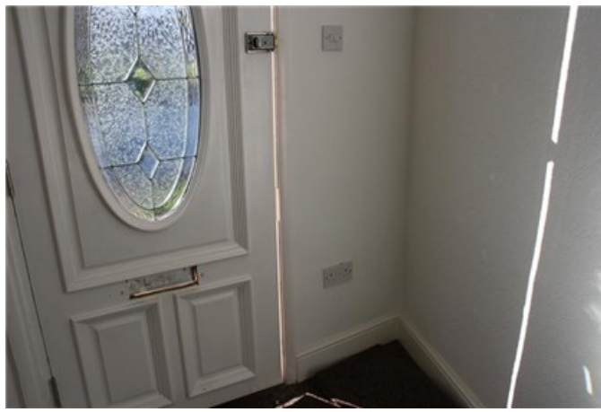
Front door will not close without force
