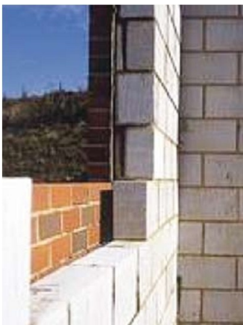
Fig1—Modern brick/block cavity wall
