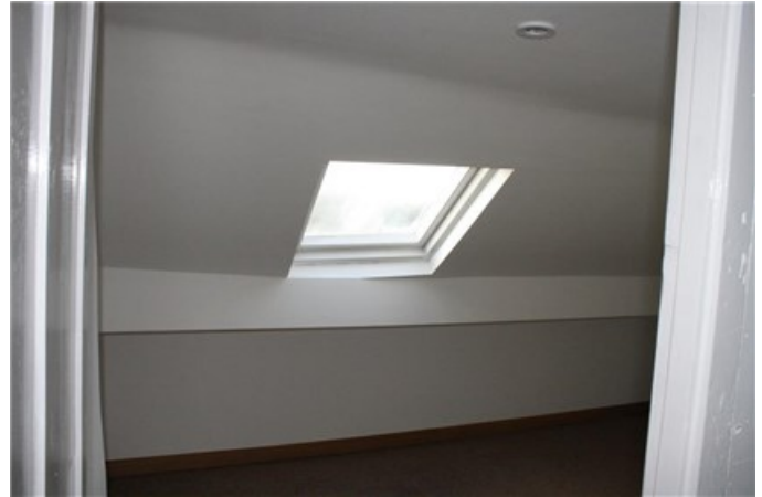
Photo of front roof room - new beam
