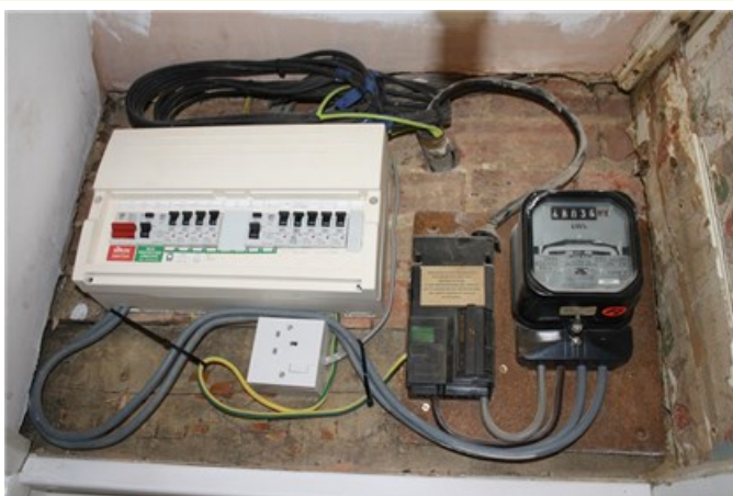
Electric meter and consumer unit
