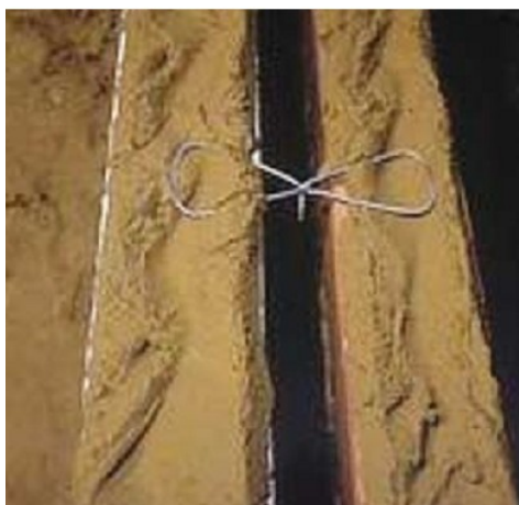
Fig2—Wall tie installation
