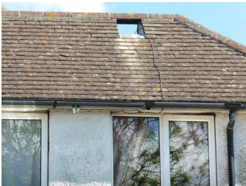
Rear roof pitch
