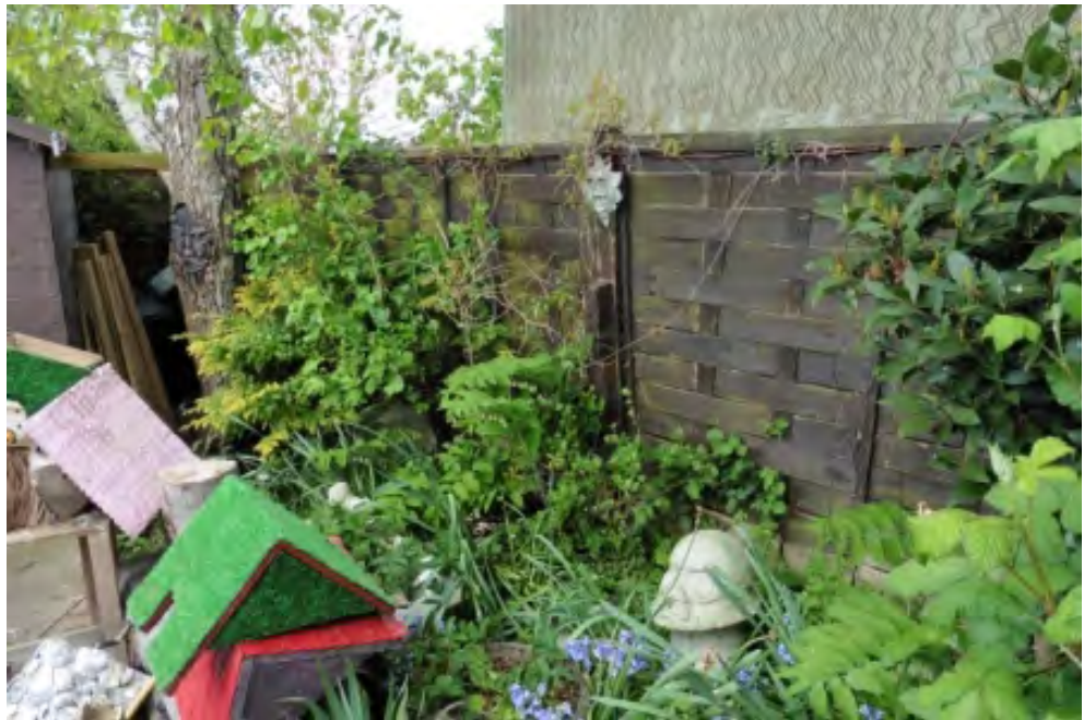
Rear boundary fencing maybe loose
